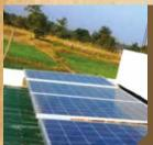
1,250 watt solar panels installed at the Foundations Community Centre in Pench. The panels supply energy to a pump and help fetch 2,100 litres of water an hour from 170 feet underground.
