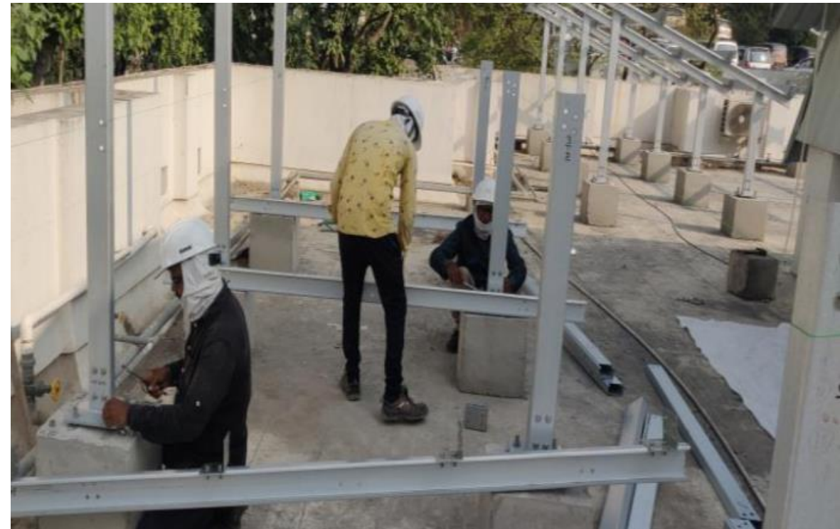
Image: Installation of panel mounting system at HV Desai Eye hospital, Pune.
